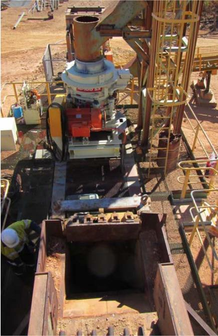
The processing plant refurbishment is nearing completion. The final major task, which is the installation of new mill bearings and the re-commissioning of the mill circuit is scheduled to be completed by the end of July 2015. The crushing circuit has been fully re-installed and tested and is operational.
