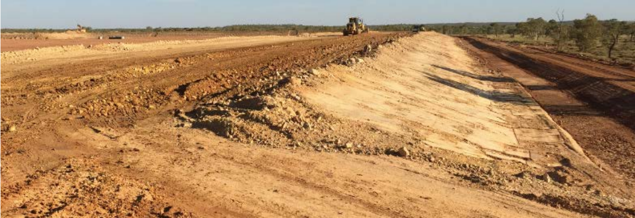
Figure 3: Tailings Storage Facility construction
