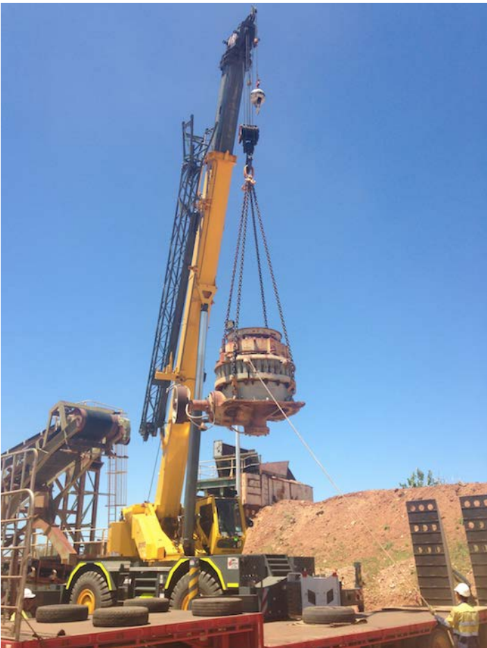
Figure 4: Removing the secondary crusher for refurbishment in Perth
