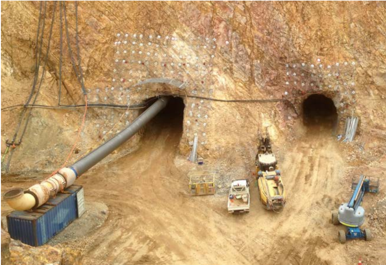
Figure 2: Portal established and development underway
