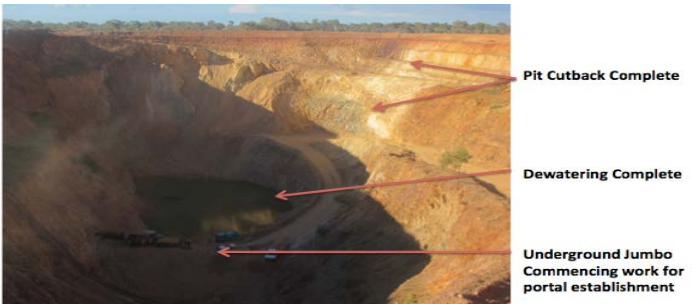
Figure 1: A comparison of the mine prior to commencement in February and approximately 1 month later on the 18 th of March.
